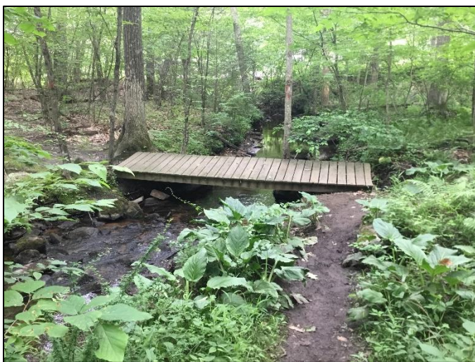
The bridge over a narrow section of Hawley Brook on the orange trail near the southern boundary is being undercut by the brook. Reinforcing the abutments and/or raising the bridge would be useful.
