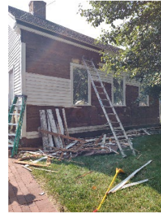
Exterior siding removed on Day 1, July 11, 2023
