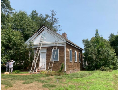
Exterior siding removed on Day 1, July 11, 2023
