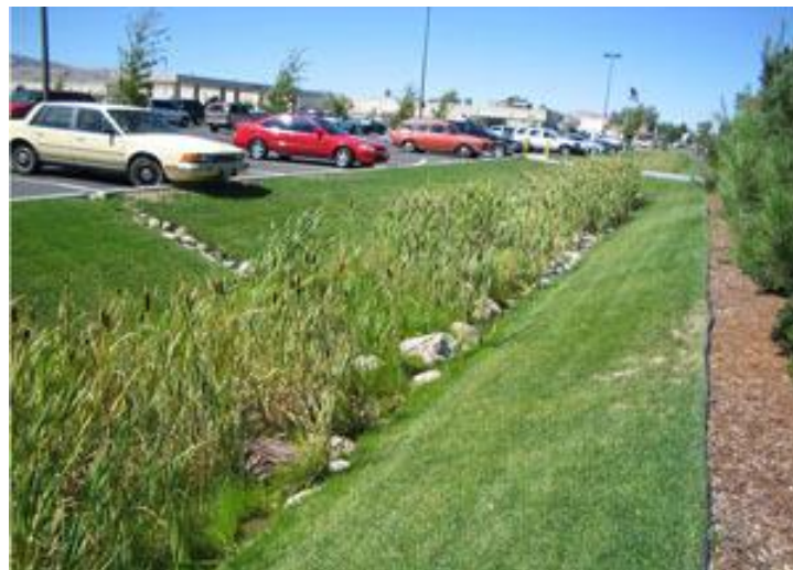
Exhibit 4-4 Vegetated Swale Adjacent to a Commercial Parking Lot
