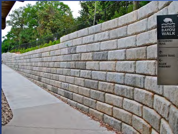
Site Retaining Wall
