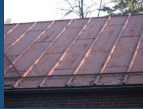
Metal Roofs, Building 1 & 2 @ 60 West Main Street
