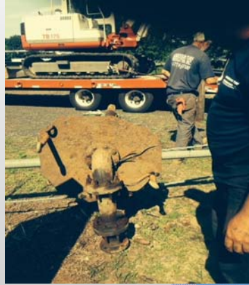
Existing piping and pump installed 1983
